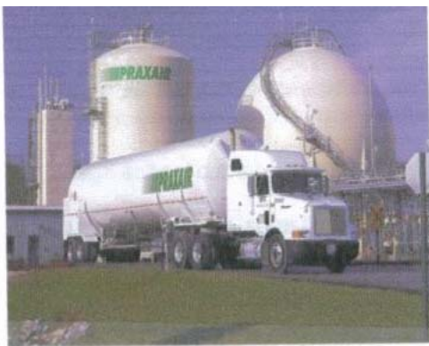
Hydrogen generation, storage and bulk distribution systems (Praxair, Inc)
